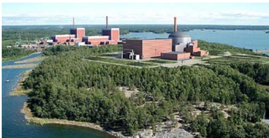
The new Finnish nuclear reactor at Olkiluoto (OLK3)
