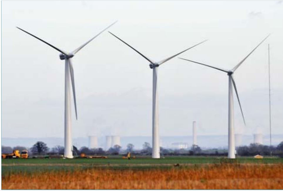
Westmill Wind Farm Co-op, Watchfield, Oxfordshire. Photo credit: http://www.energy4all.co.uk .
